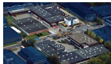
NORD gear factory Glinde
