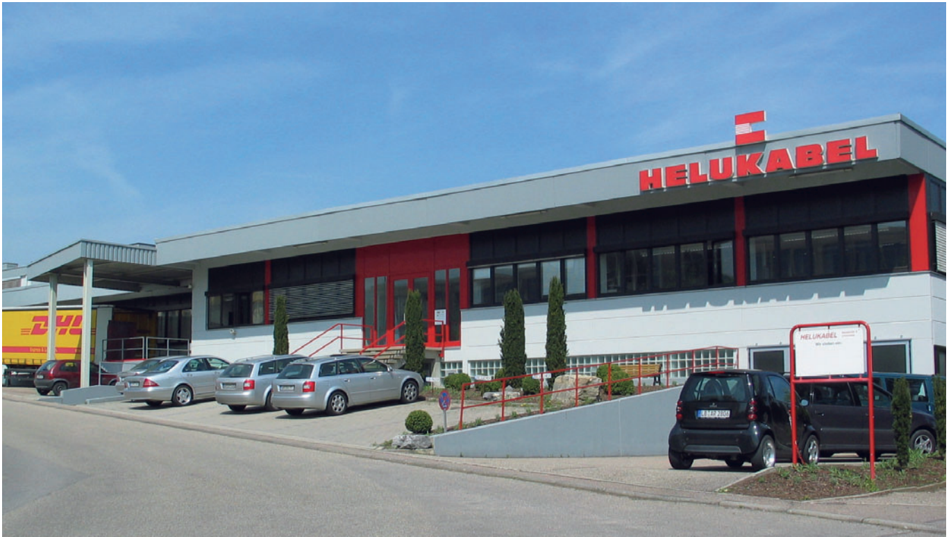
Photo: HELUKABEL® – Headquarters Hemmingen
