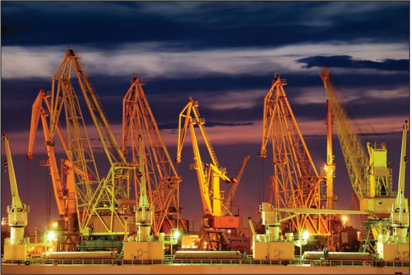
Overhead Crane Applications
